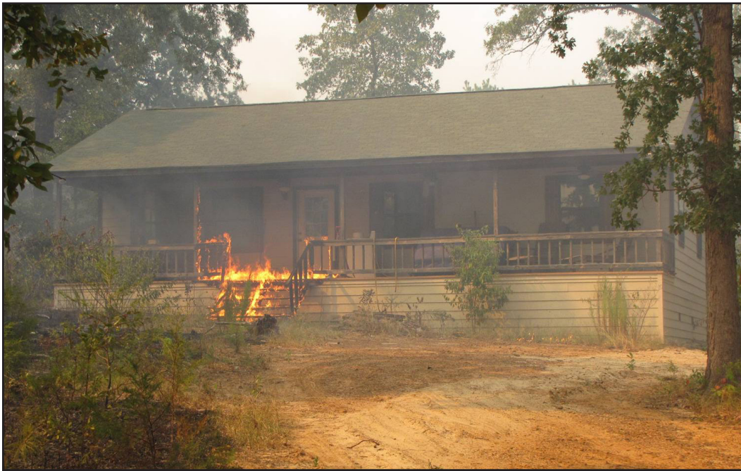
Relatively fire-resistant homes can ignite during low-intensity wildfires if a path of combustible material, such as stairs or support beams, leads the fire up to the home.
