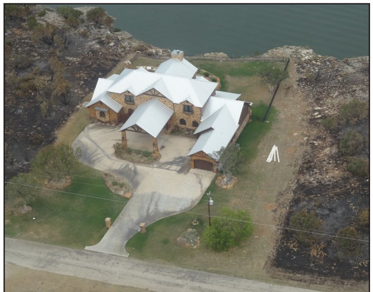
This home with fire-resistant construction and landscaping survived the Possum Kingdom Complex.
