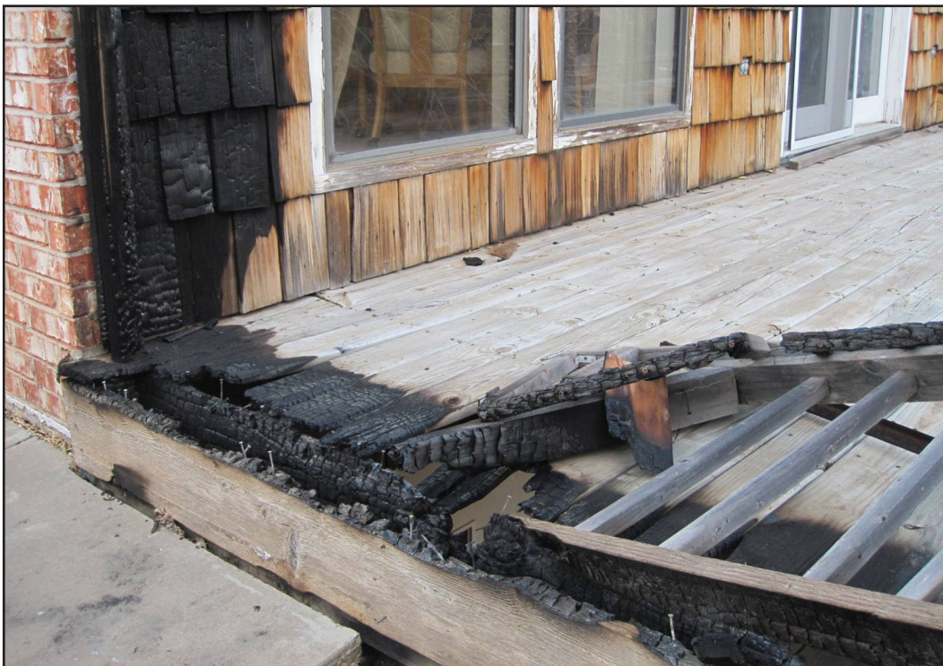
Combustible decks that aren't treated with fire-resistant paint or chemicals are more likely to catch fire.
