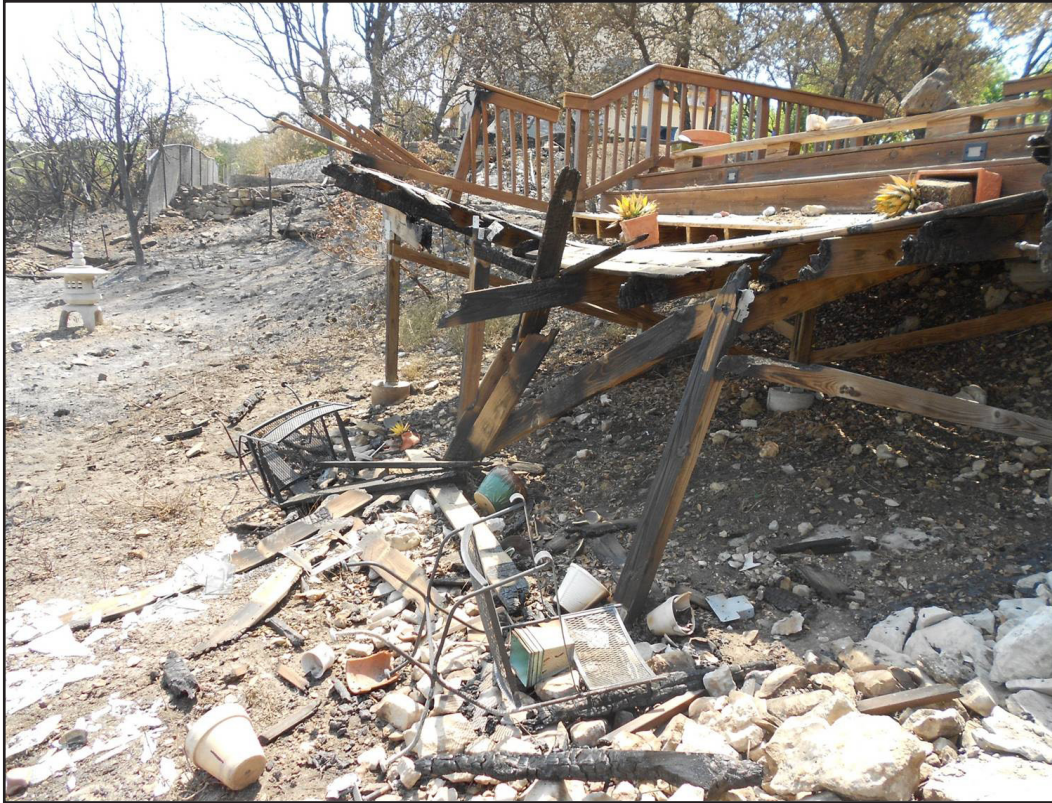
Combustible materials on and around decks can increase the chances of ignition.
