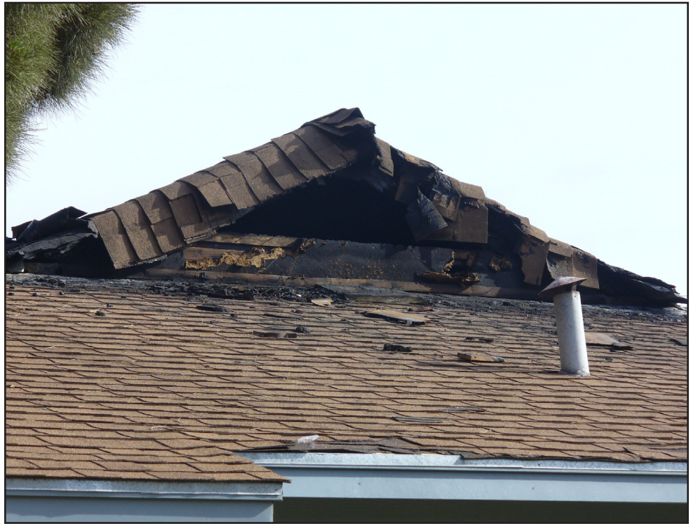
Even though this home had non-combustible roofing, embers from the Hickman Fire ignited the attic days after the blaze passed through town.
