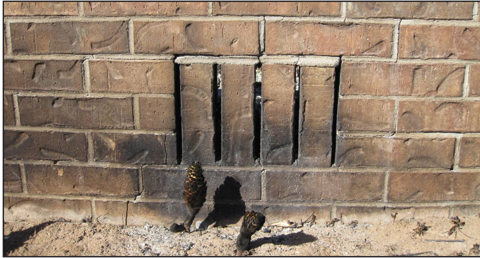
Open or unscreened foundation vents provided embers access to a vulnerable pier and beam foundation.
