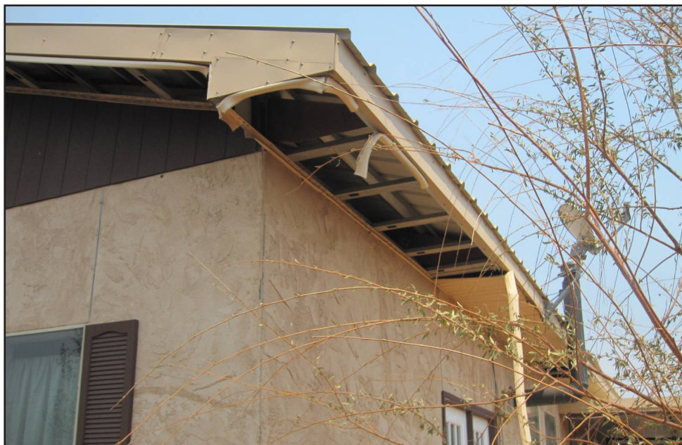
Combustible soffits can melt or ignite, giving embers access to an attic. Once inside, the embers can go undetected until it is too late to save the home.
