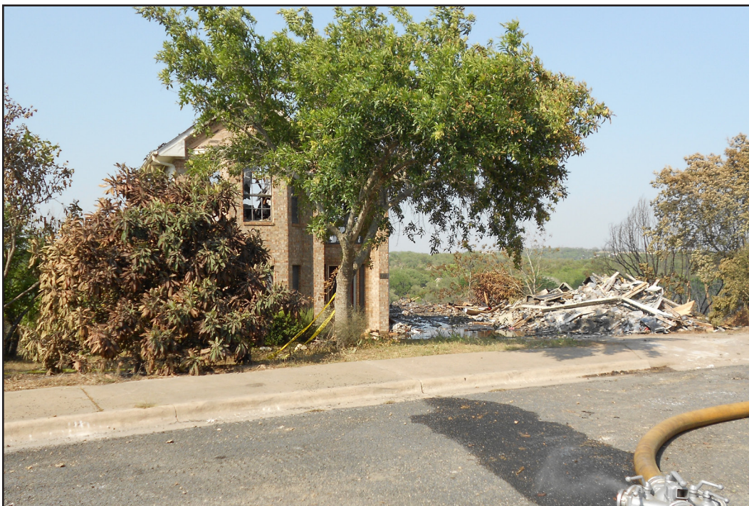
This photo shows an example of structure-to-structure ignition. Note the unburned vegetation surrounding the home, which indicates ground fire intensity was low and points to ember intrusion as a probable factor in ignition.
