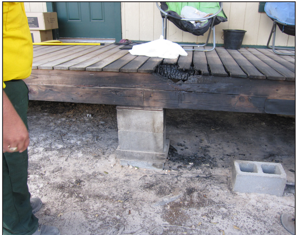
The porch of this home on the Dyer Mill Fire was ignited by embers that were spread by strong winds. Fortunately, a fire engine was stationed near the home and firefighters were able to extinguish the blaze before it spread to the house.
