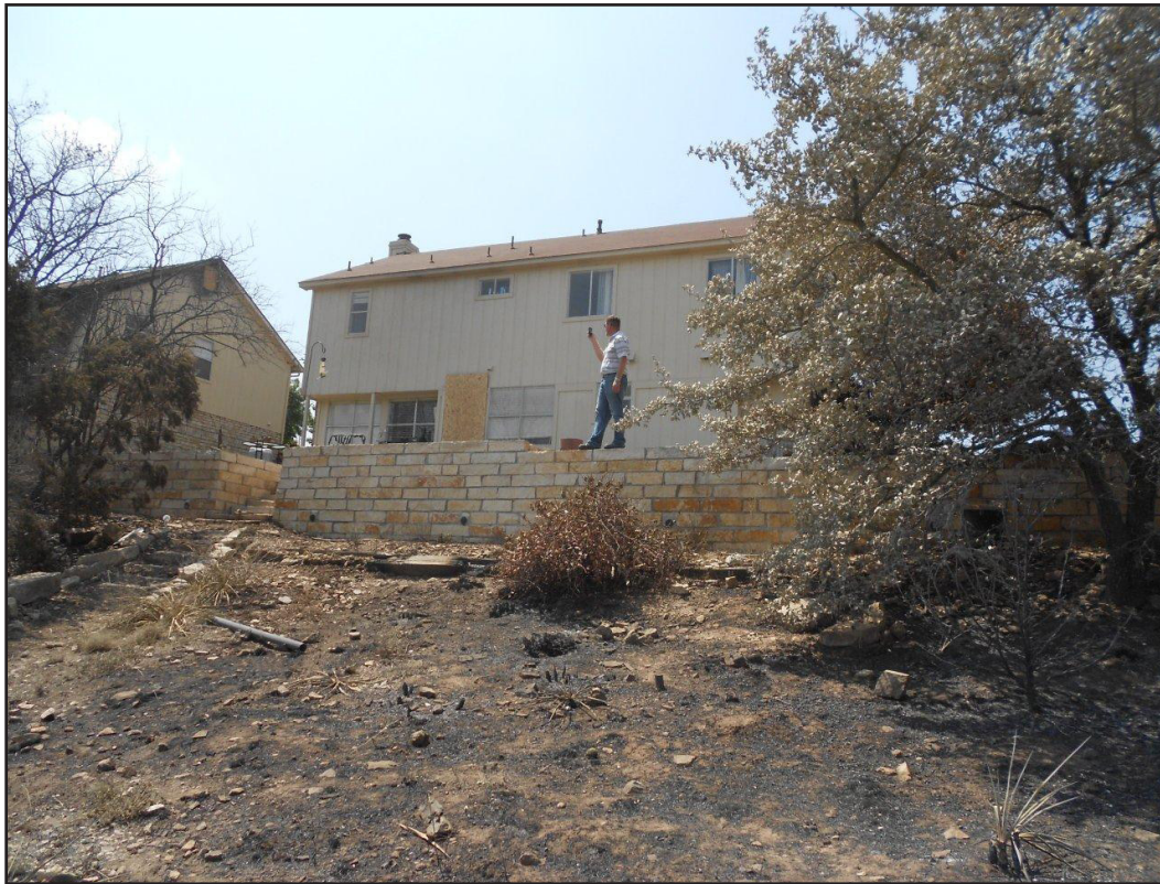
The noncombustible brick retaining wall along the back of this home helped stop the spread of the Pinnacle Fire. Conversely, retaining walls constructed out of combustible materials such as railroad ties can ignite easily and burn intensely for long durations.
